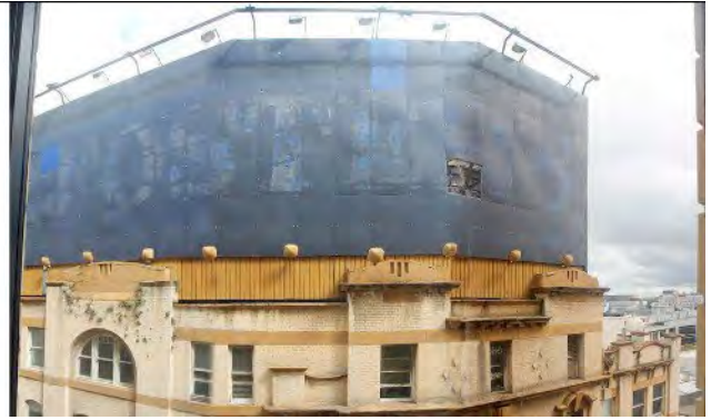
Existing situation – view from adjoining hotel
